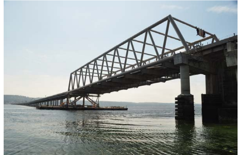
New Hood Canal Bridge
